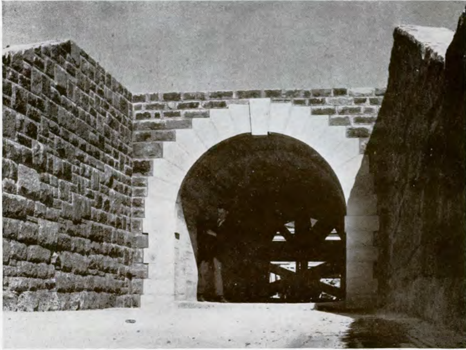
Brushes Floodwater Tunnel
