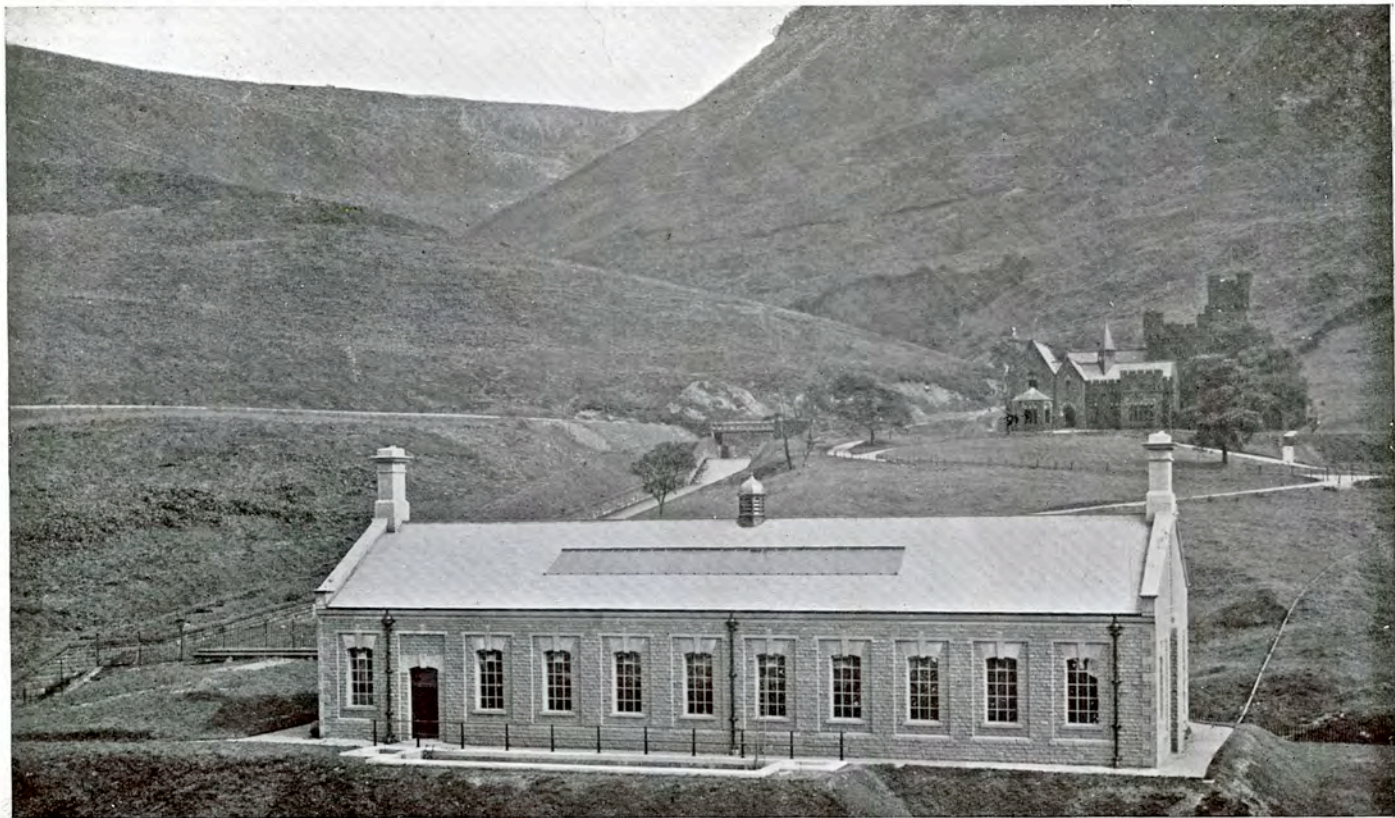
ASHWAY GAP FILTER HOUSE
