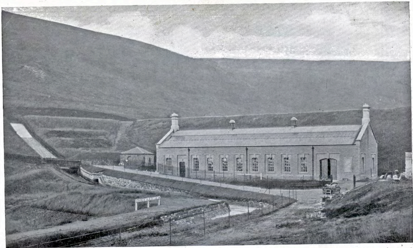
BRUSHES FILTER HOUSE
