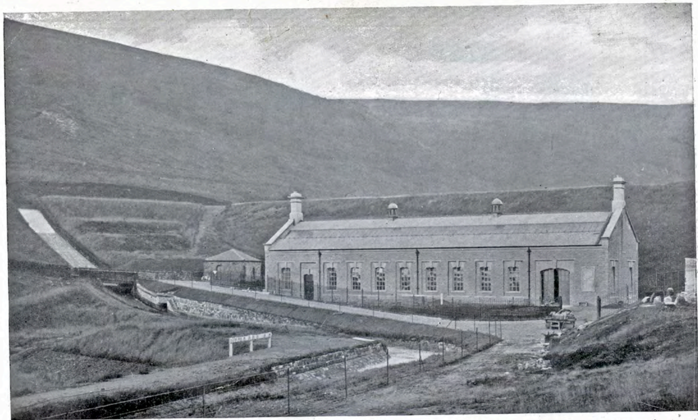
BRUSHES FILTER HOUSE
