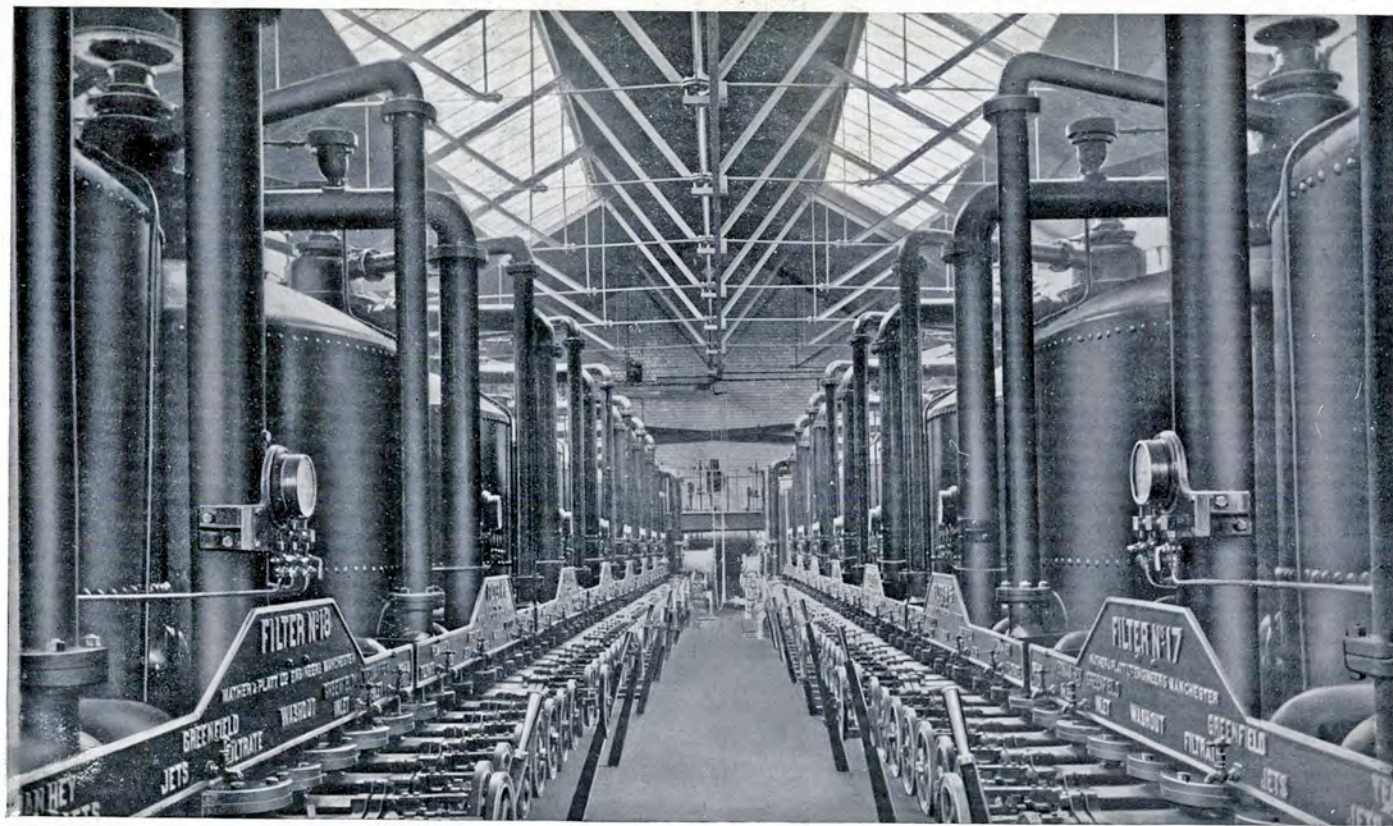
ASHWAY GAP FILTER HOUSE
