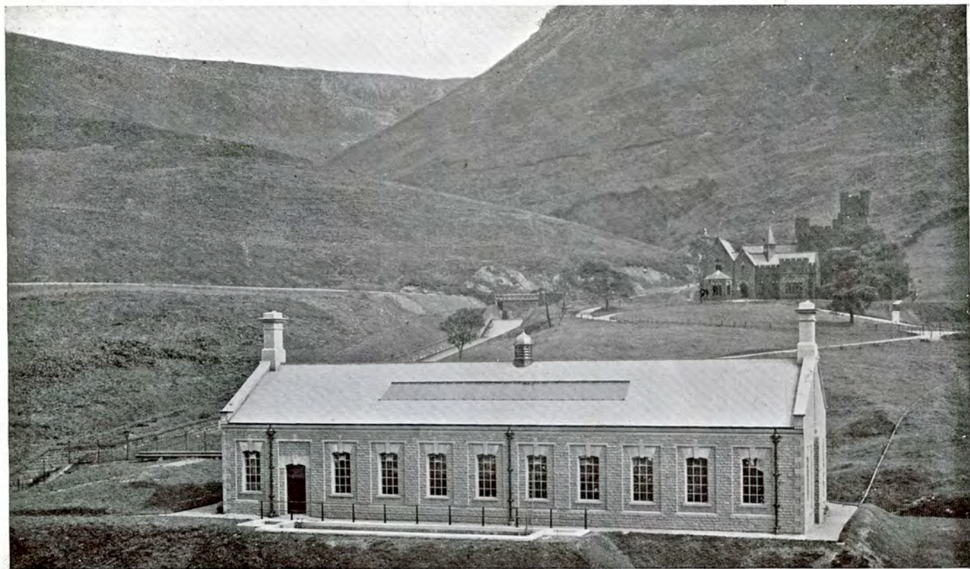
ASHWAY GAP FILTER HOUSE
