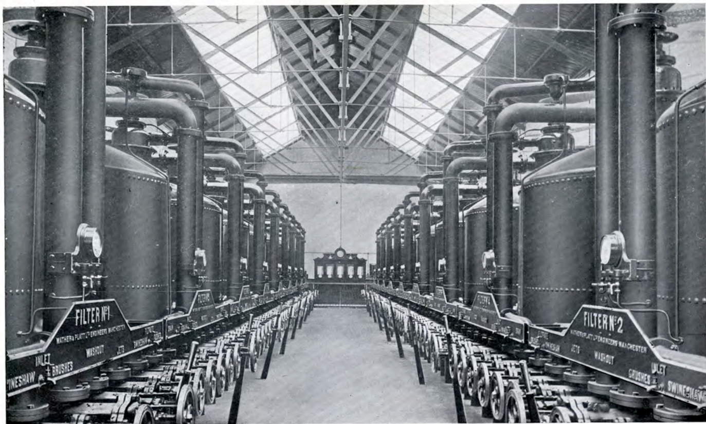
BRUSHES FILTER HOUSE
