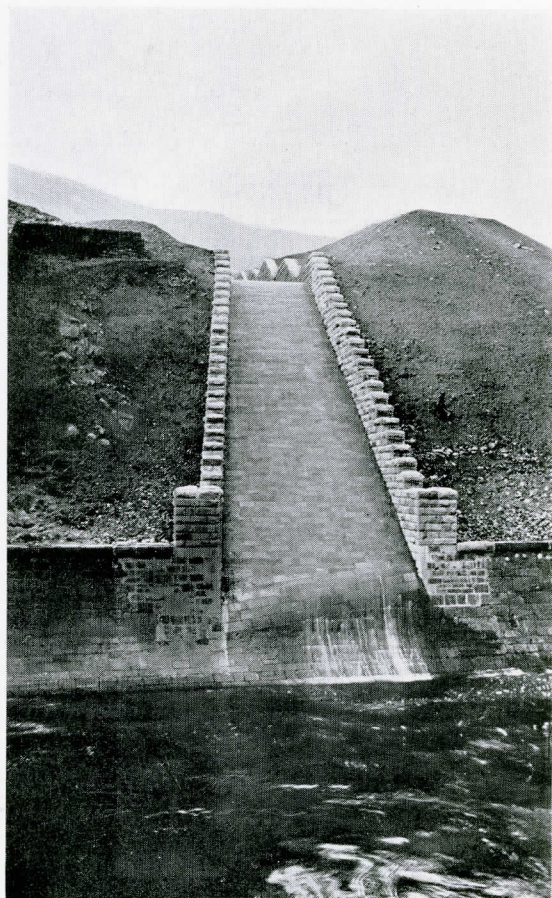
MASONRY CHUTE AT GREENFIELD BROOK.
